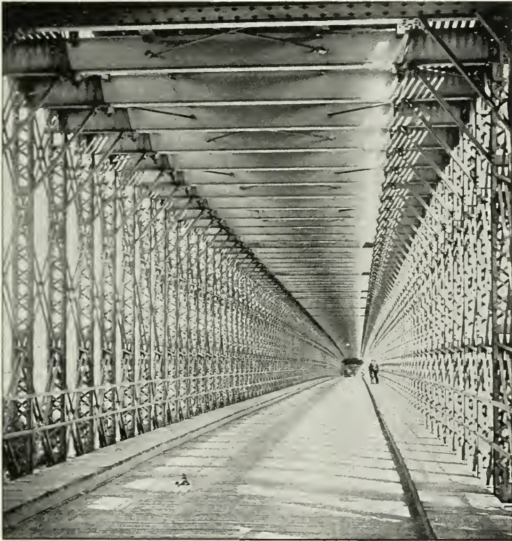
SUSPENSION BRIDGE ROADWAY.
